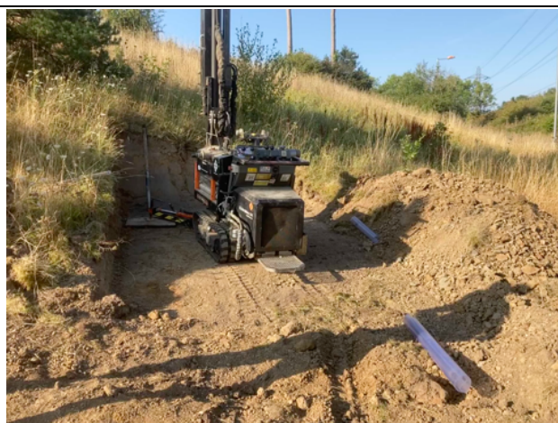
Slope levelled to enable window sampler at WS1. The ground level at the window sample position was reduced by approximately 1m.
