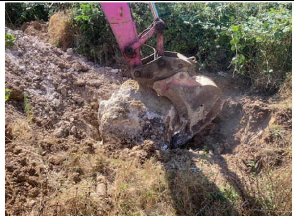
Concrete obstruction being removed from location of WS2
