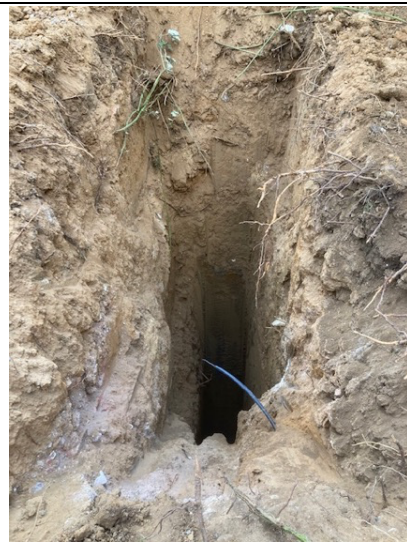
Location of WS3 following excavation of concrete obstruction
