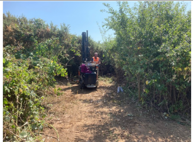
Vegetation cleared to give access to WS3
