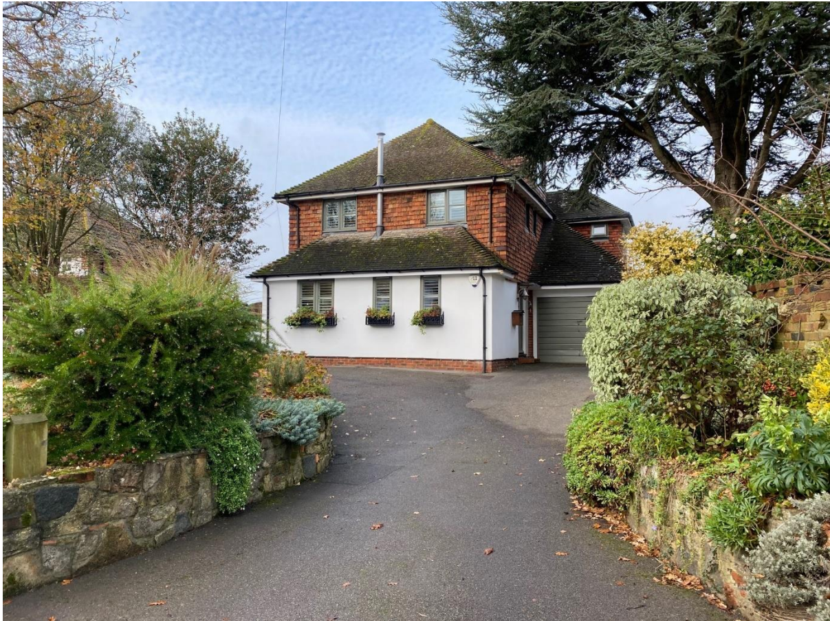
Photograph 1 – North West Elevation
