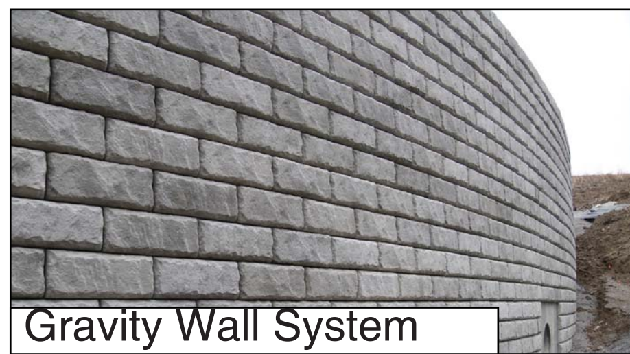
Gravity Wall System
