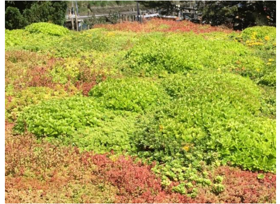
Extensive sedum roof
