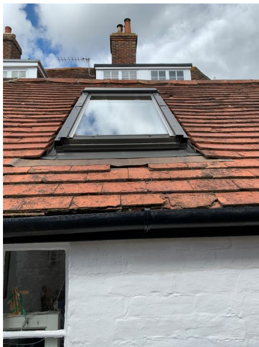
Rooflight to rear roof
