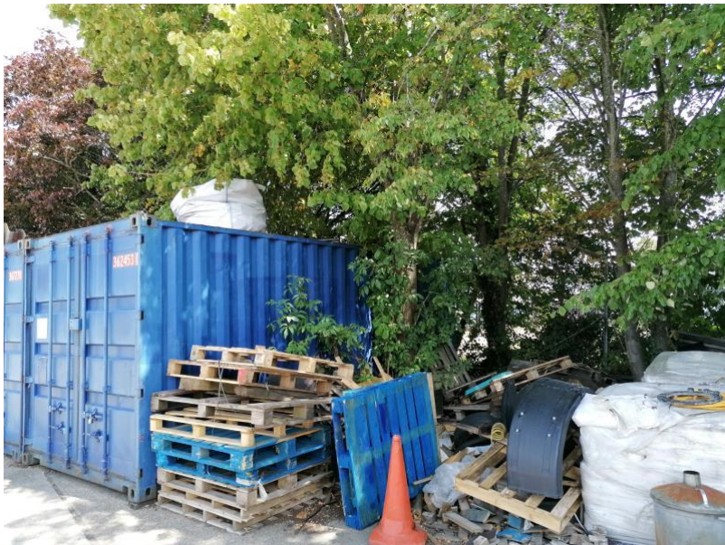
Photo 5: Further views of material storage amongst trees on site.
