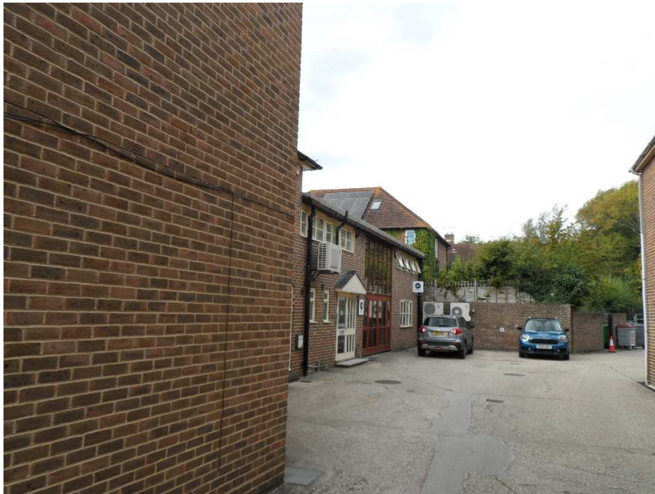
6 – Front of business units to east
