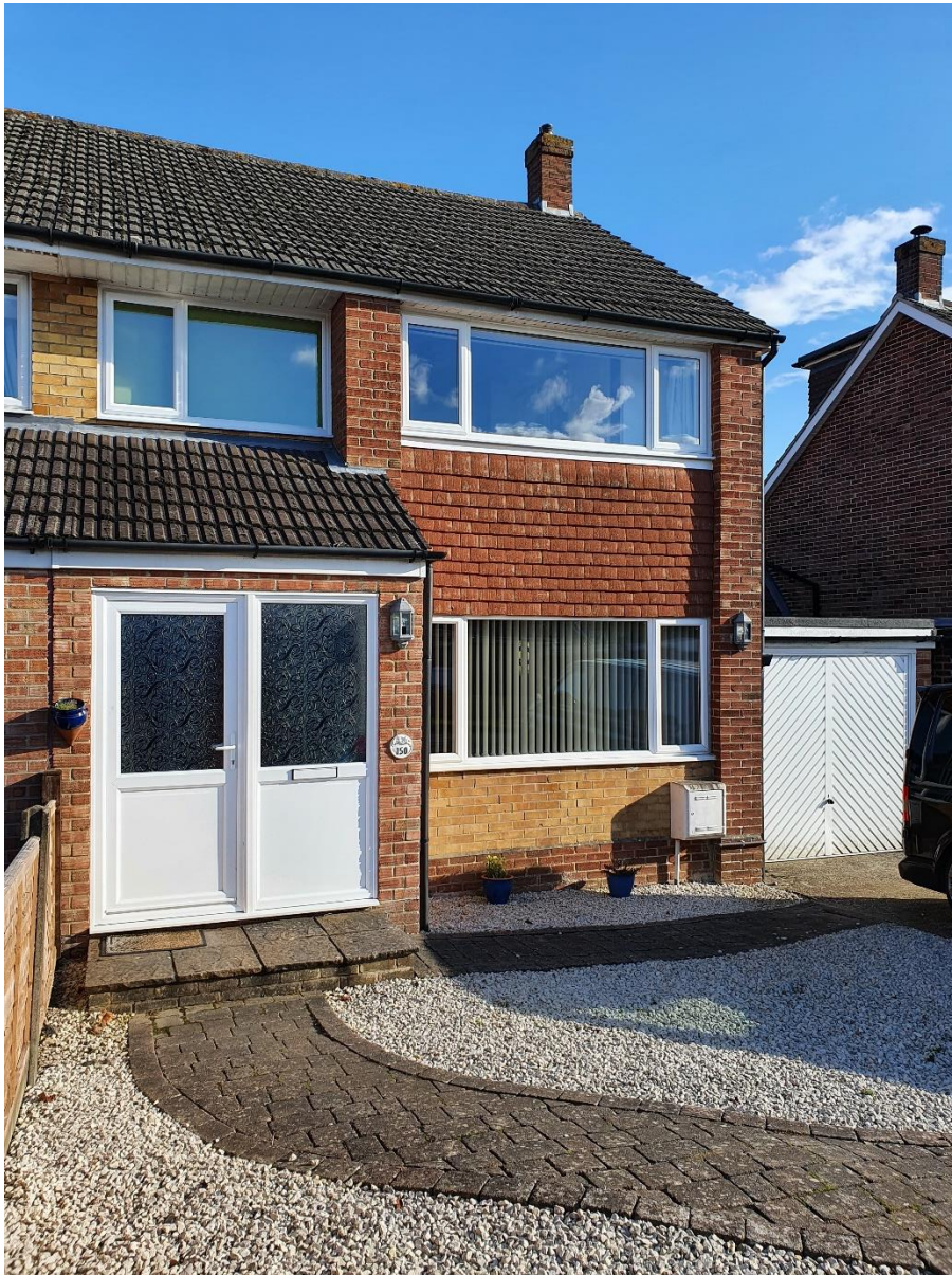
APP/20/00776 – 150 Greenfield Crescent Site Photos
