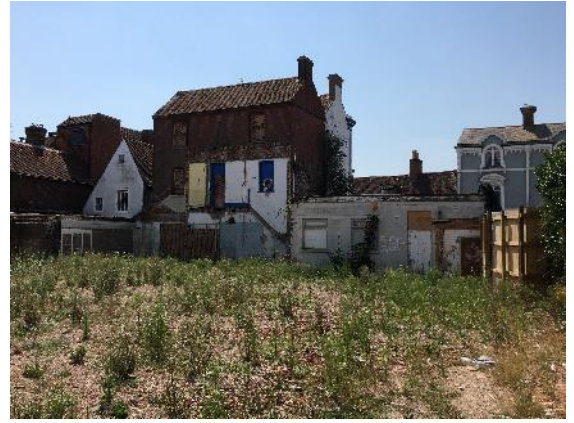
Photograph 2. Rear elevation of No. 9 (to right) with land behind No. 13 in foreground.
