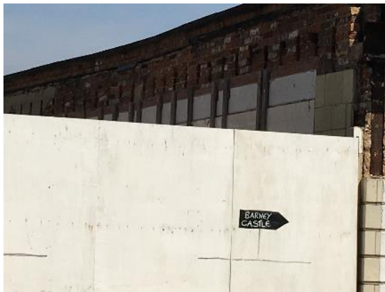
Photograph 7. Gaps in No. 9 where neighbouring building (No. 7) has been demolished
