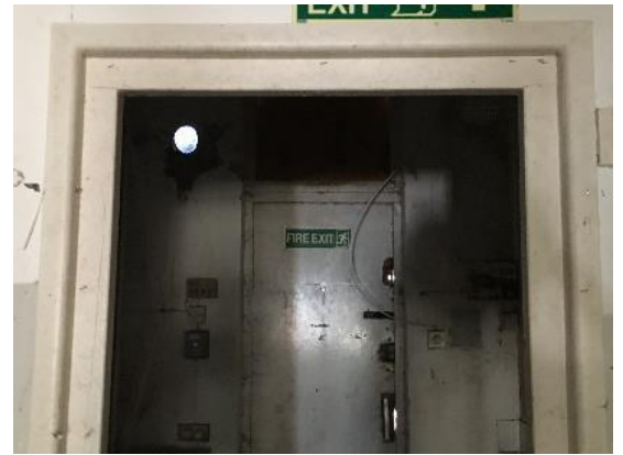
Photograph 6. Open hole from removed extractor unit at the rear of No. 9 East Street
