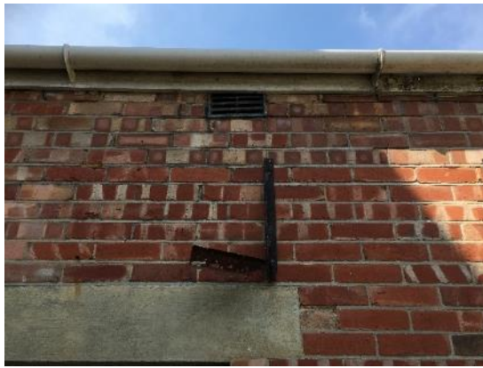
Photograph 5. Air vent to No. 9 East Street
