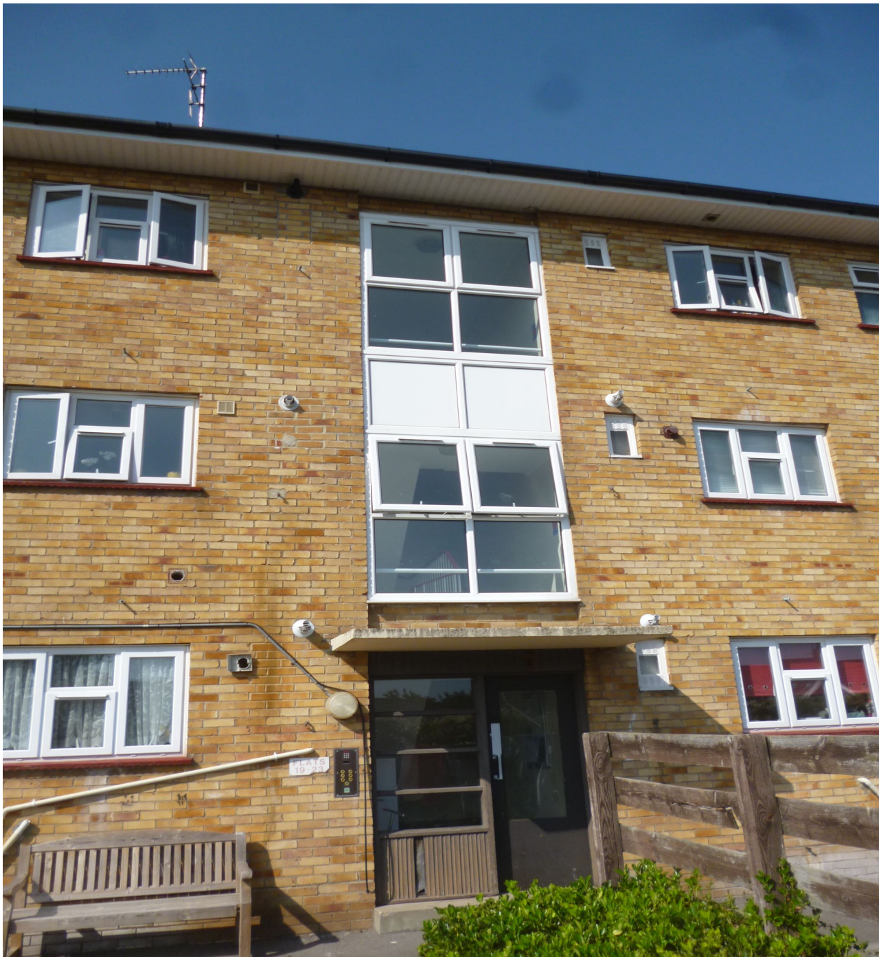
Existing Rear Elevation Image
