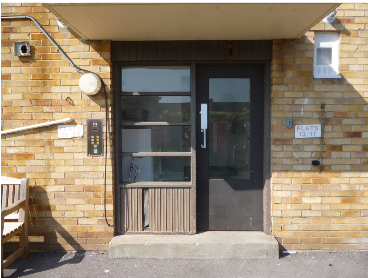
Existing Rear Door B Image
