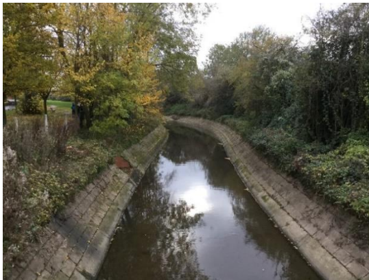
Photo 11: immediately downstream of the confluence with Riders Lane Stream (OSNGR SU 71029 07447).
