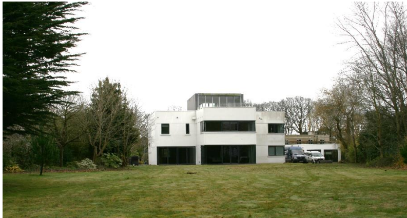
Northshore – number 40 Sinah Lane – Existing house on the site
