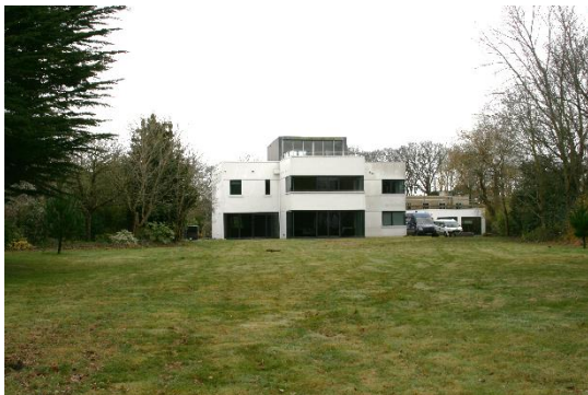
Northshore – number 40 Sinah Lane – Existing house on the site
