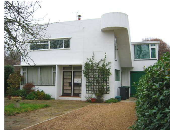
The White House – number 44 Sinah Lane – designed by Connell, Ward and Lucas 1934
