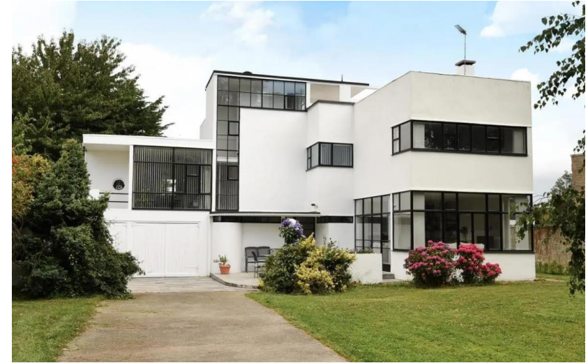
The Saltings – number 42 Sinah Lane – designed by Connell, Ward and Lucas 1934
