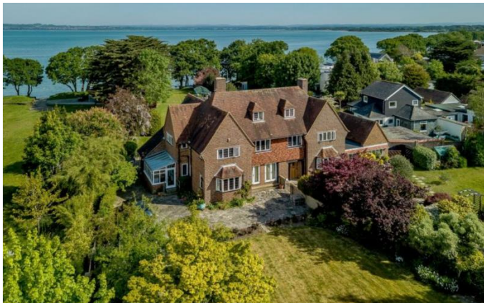
38 Sinah Lane – Traditional Arts and Crafts house located to the east of the site
