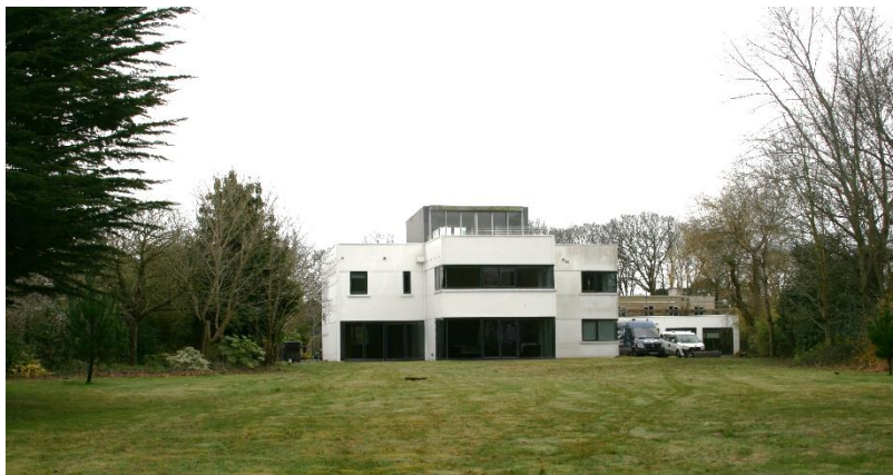
Northshore – number 40 Sinah Lane – Existing house on the site
