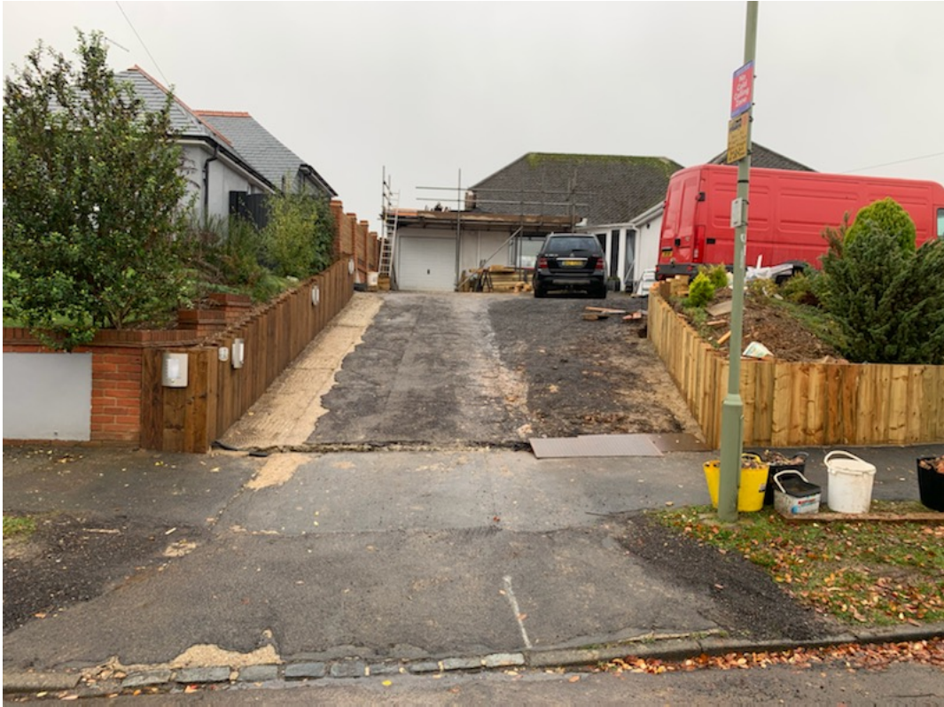
The front elevation of the appeal subject.
