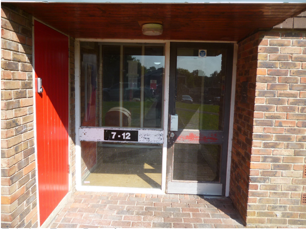
Existing Front Door Image
