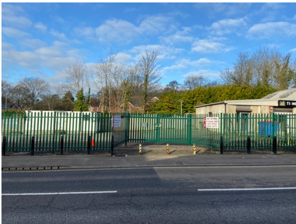
The access gates to the site, via London Road.
