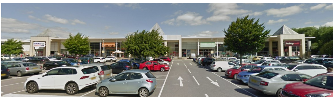
VIEW OF UNITS 1 to 7 FROM THE SOUTH
