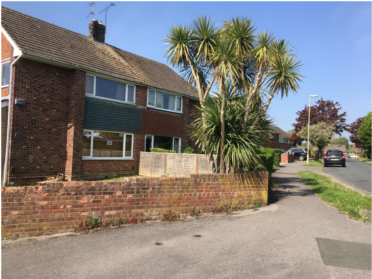
Photo 10: Front of house looking towards No. 14 Elderberry Way from road corner
