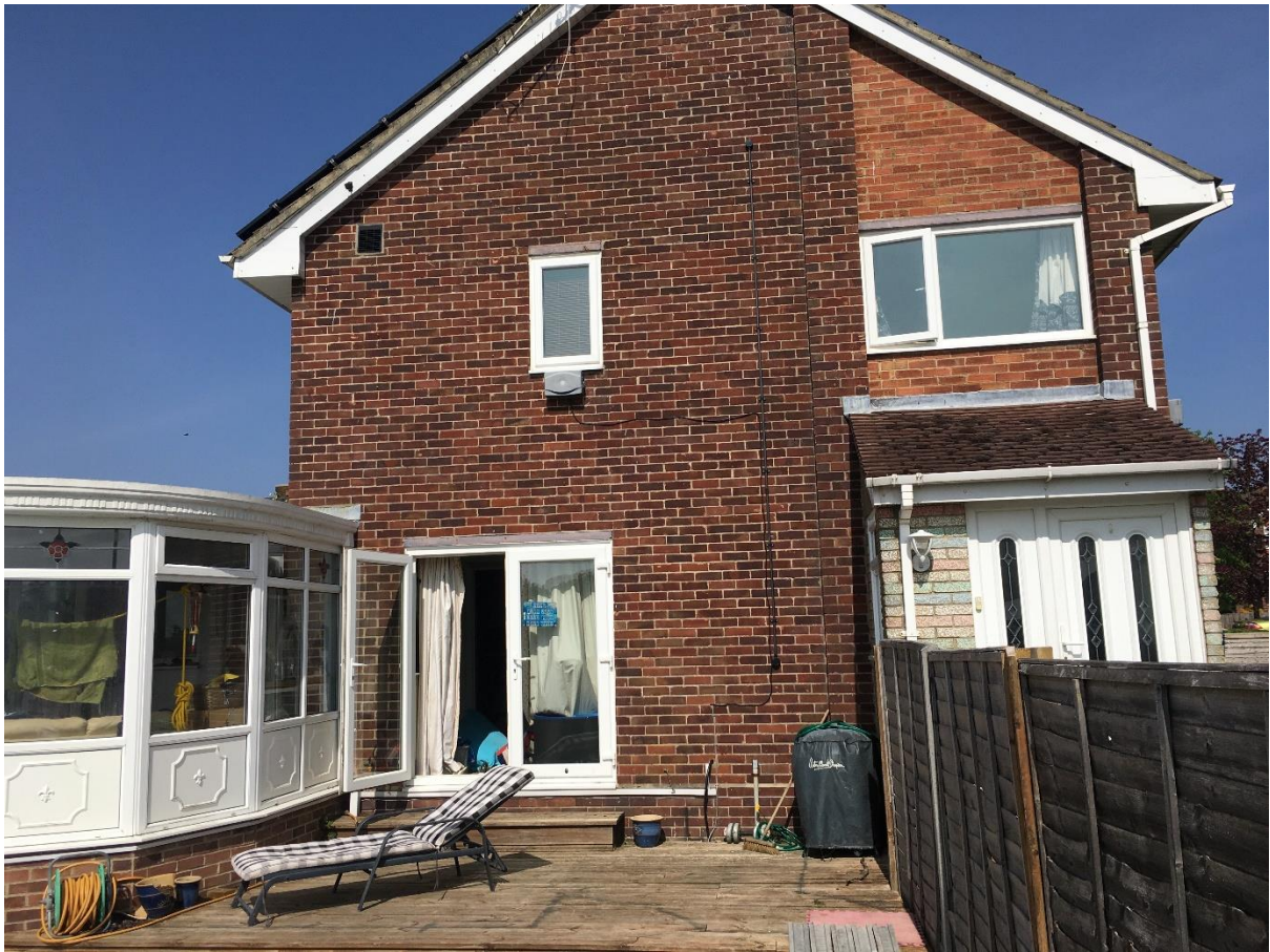
Photo 4: Side of House from back garden boundary wall
