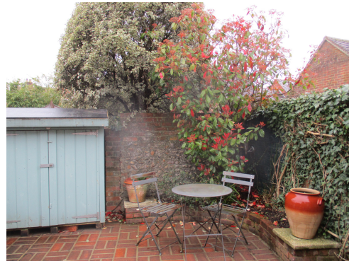
Fig 6 – View of rear wall (flint/brickwork) and boundary wall with No. 12 (brickwork but covered with ivy)
