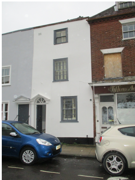
Fig 1 – Front view of property from Queens Street.
