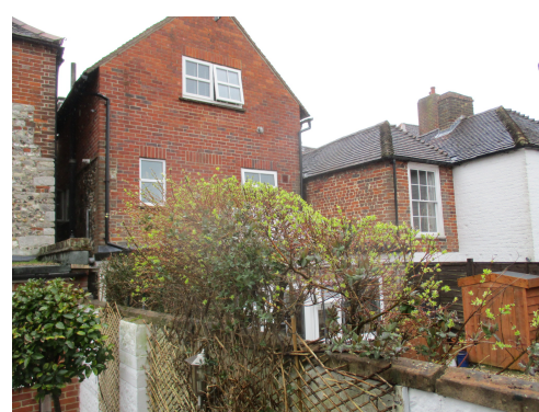
Fig 8 – View of painted blockwork boundary wall with No.8, looking back towards the rear of the dwelling standing on upper terrace.
