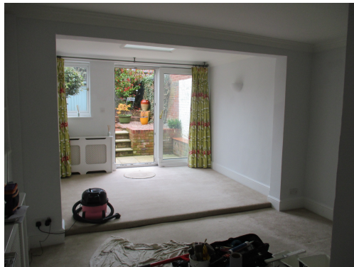
Fig 3 – View of existing single storey extension showing raised step up and existing opening from the original dwelling.
