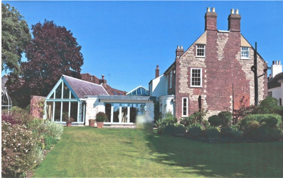
Photo 05 Saxted House glazed extensions
