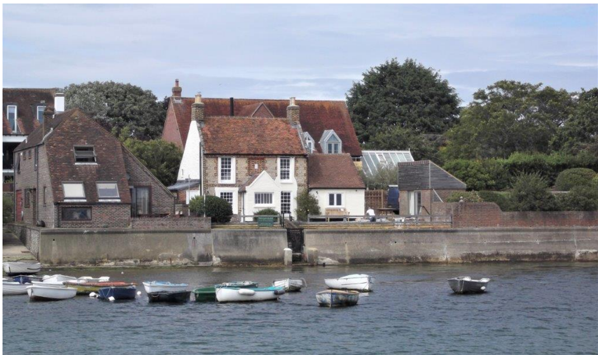
Photo 07 – showing the roof and conservatory to Tower House in the distance
