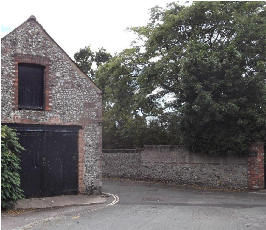
Photo 04 – Adjacent the site access to the application site
