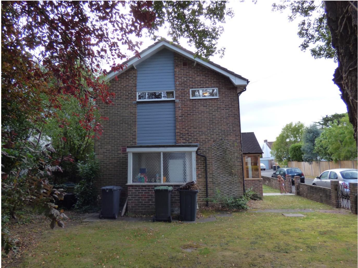
Photo 4: Side of the property where the extension would be
