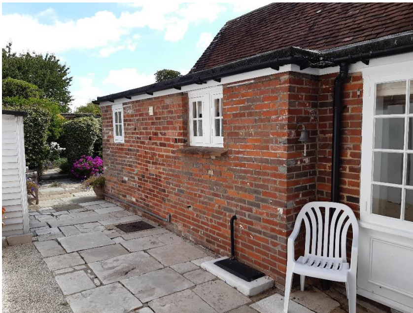
Figure 6: External Wall of WC, 2020
