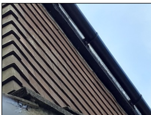
Figure 5 – tight fitting hanging tiles on the southern elevation of the dormer window
