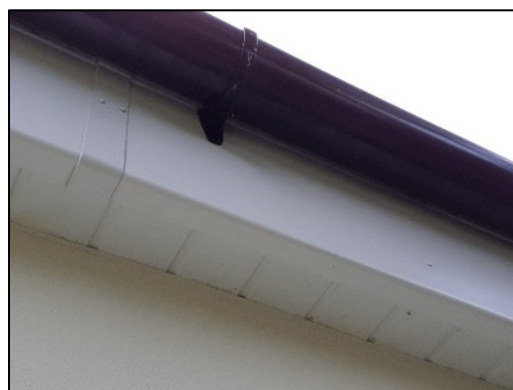
Figure 5 – plastic underboards on the eastern elevation of the extension
