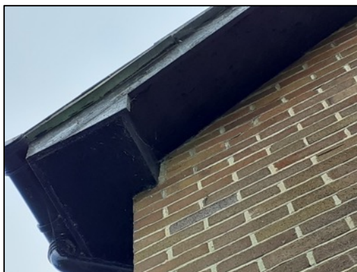
Figure 3 – wooden underboards on the northern elevation of the original house
