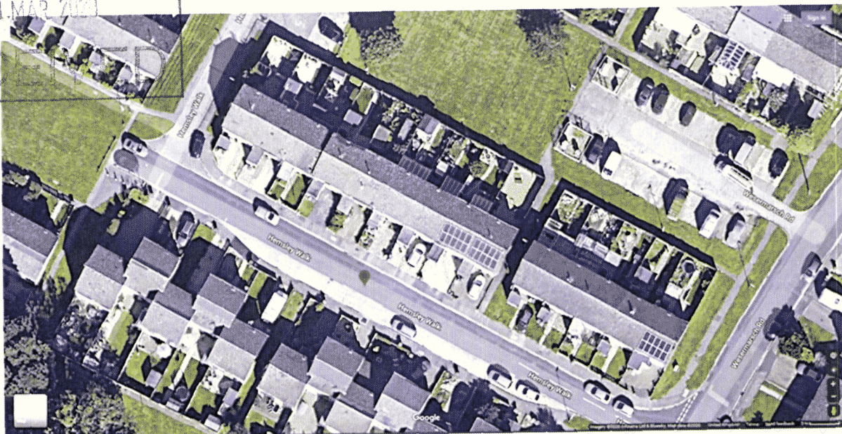
Photograph taken from Google Maps showing flat roofs in Hemsley Walk, prior to development.
