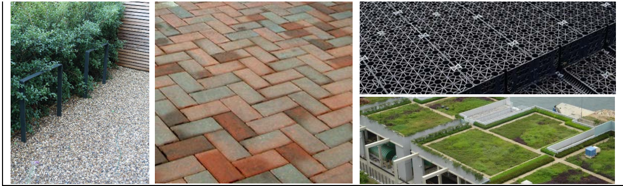
Figure 1: Surface water storage facilities and potential SuDS features - rainwater harvesting, on-site tank storage, rain garden soak-away and green roofs. (Source: UK SuDS Manual)
