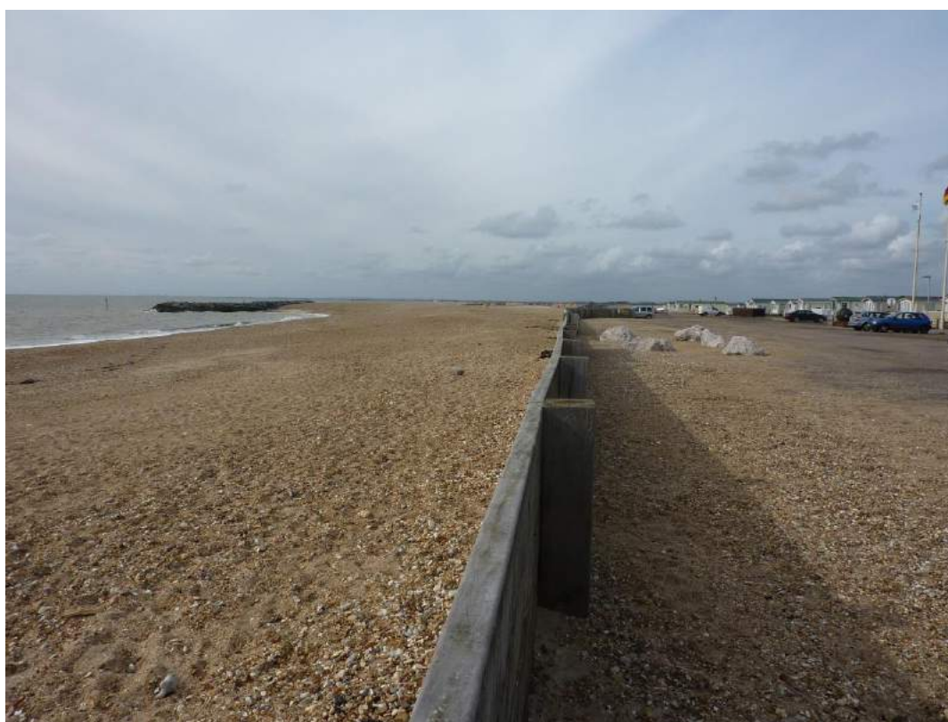
Figure 1-3: Wide shingle beach and rock groynes at Bunn Leisure complex
