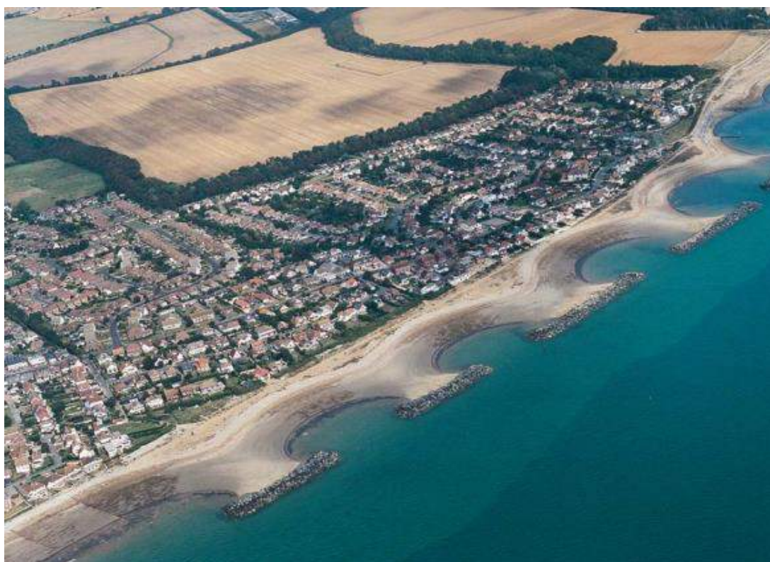
Figure 1-6: Elmer coastal defence and beach management system (image courtesy of South Downs Coastal Group)
