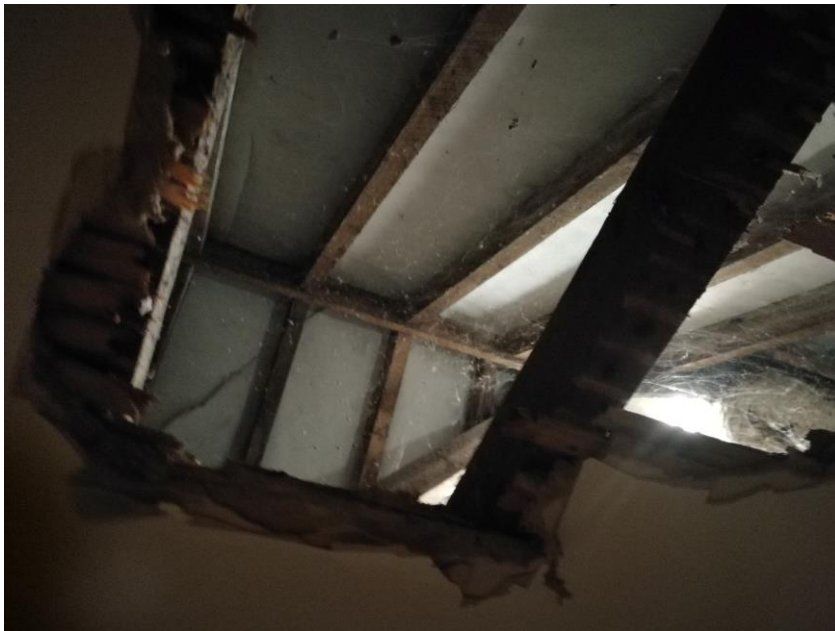
Photograph 14: View of roof void with dense cobwebs visible
