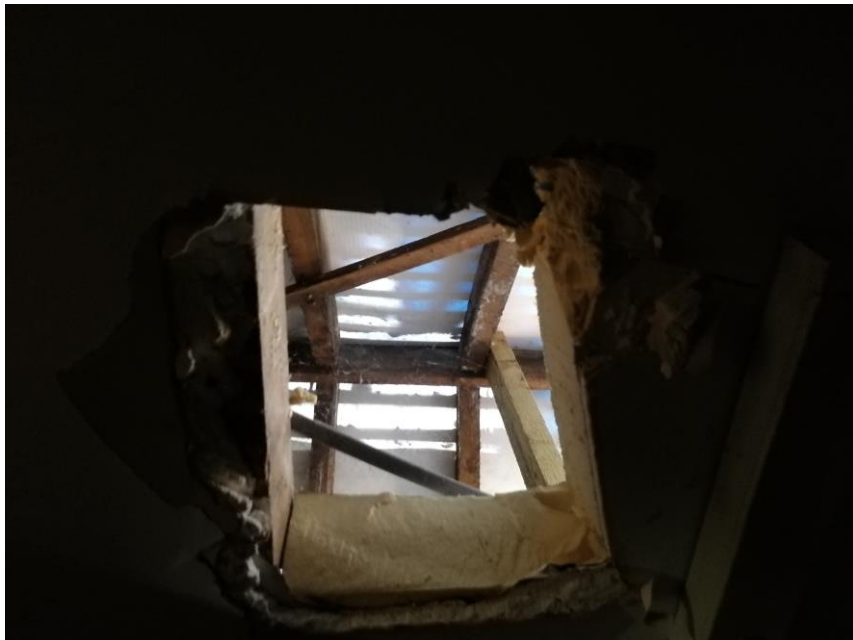
Photograph 12: View of roof void of small pitched roof extension via a hole in ceiling. Examined via ladder and no evidence of bats recorded
