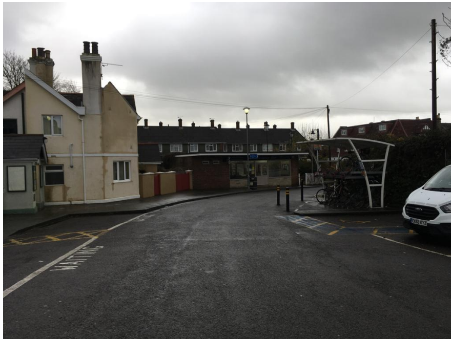
Figure 2: Station access road looking towards North Street
