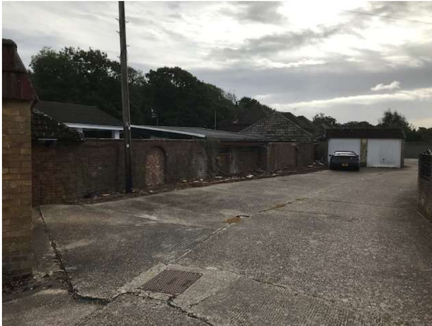
Fig.14 – Photograph taken from the entrance to garage Block A (right) looking east towards the buildings at Sparshatts of Havant.
