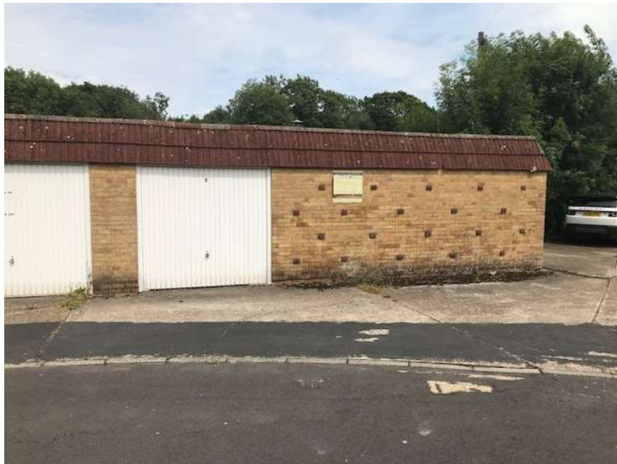
Fig.13 – Photograph taken from Willowdene Close looking east towards the front elevation of garage Block B with the entrance to garage Block A (right)
