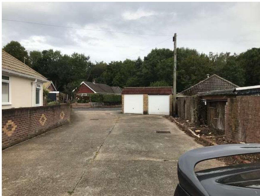
Fig.5 – Photograph taken from within the site looking north-west towards the end elevation of garage Block B, entrance to garage Block A (left) and the side elevation of 8 Willowdene Close (far left).
