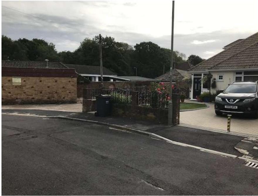
Fig.4 – Photograph taken from Willowdene Close looking north-east towards the entrance to garage Block A with the end of garage Block B (left) and 8 Willowdene Close (right).
