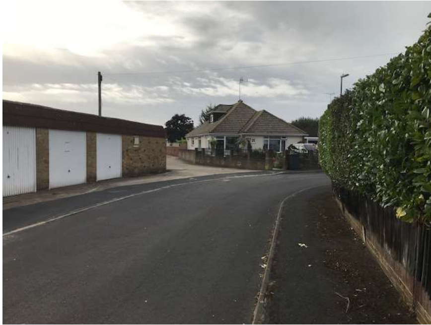
Fig.2 – Photograph taken from Willowdene Close looking south towards the entrance into garage Block A with Block B (left) and the bungalow at 8 Willowdene Close (centre).
