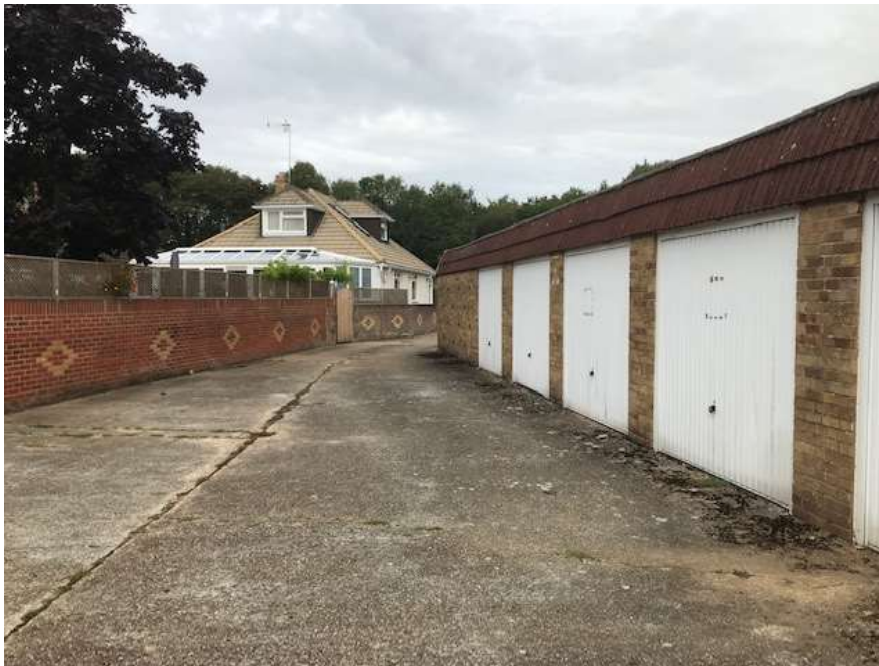
Fig.9 – Photograph taken from within the site looking north-west with garage Block A (right) and 8 Willowdene Close (left).
