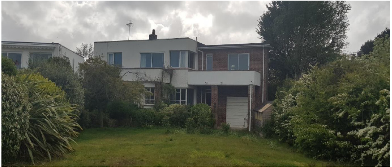
View of the Eastern elevation, which faces towards the foreshore of Hayling Island
