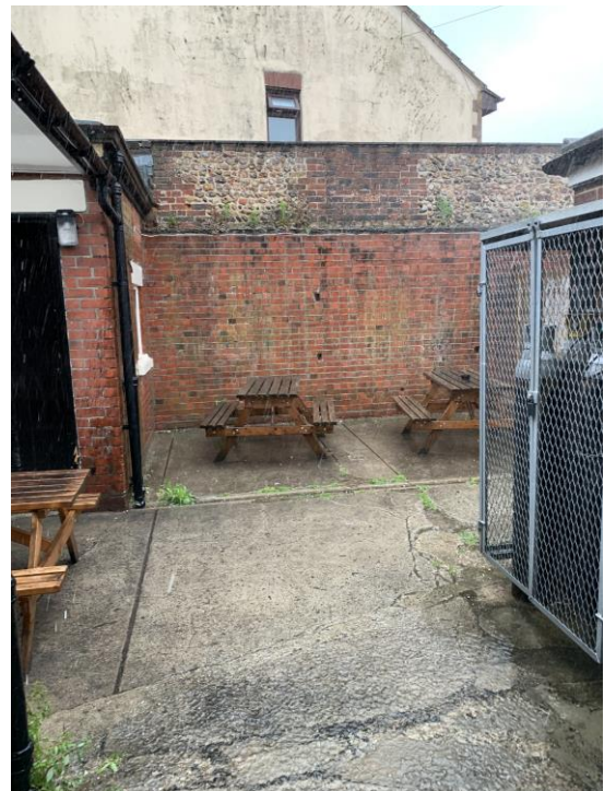
Fig F. Existing Garden – view of rear wall
