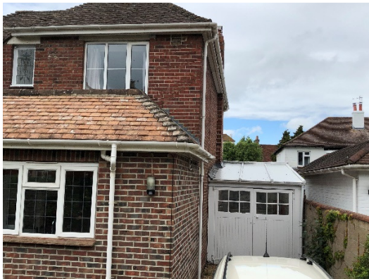
Figure 1, existing garage to be demolished and re-built.
