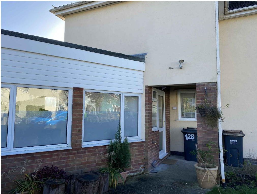
View upon arrival as existing; differing scales, materials and lack of clear entrance. Lack of privacy and security through historic space planning and various access points.
