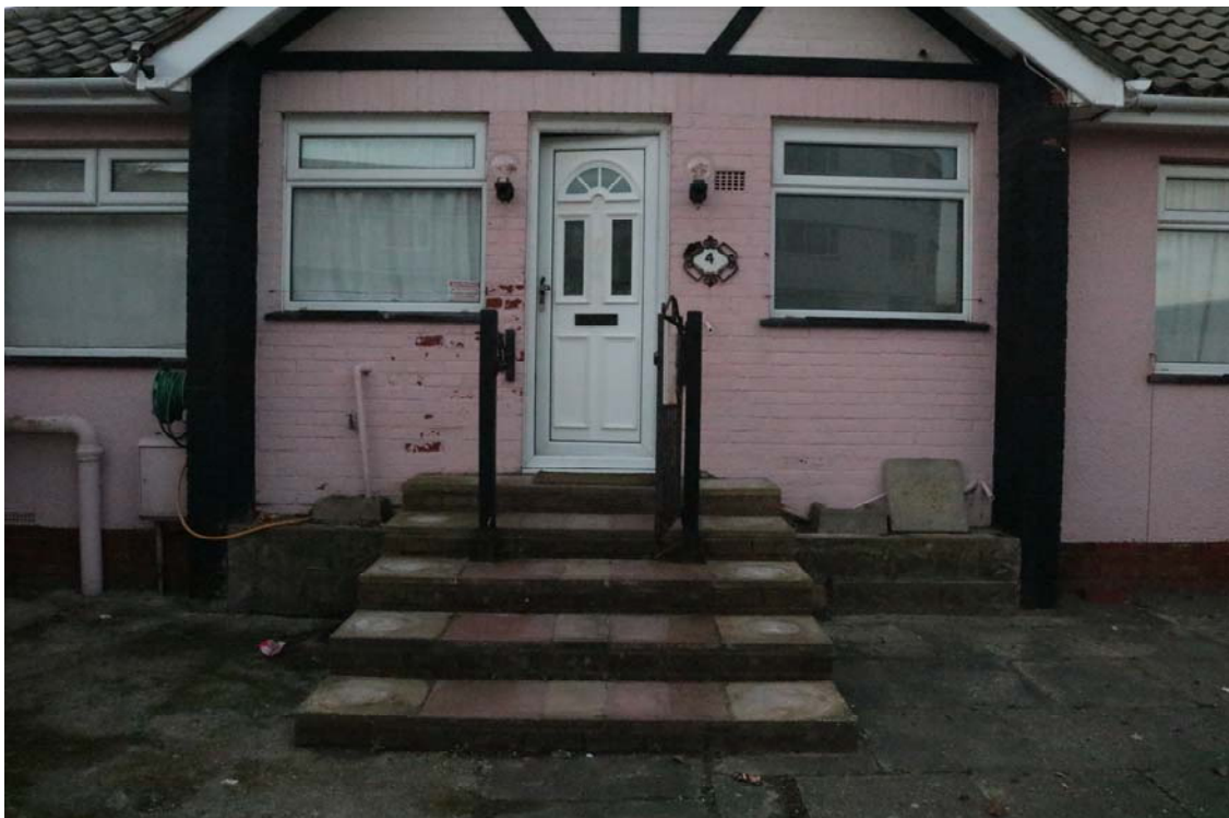
Photograph showing steps and dpc level to existing bungalow.
