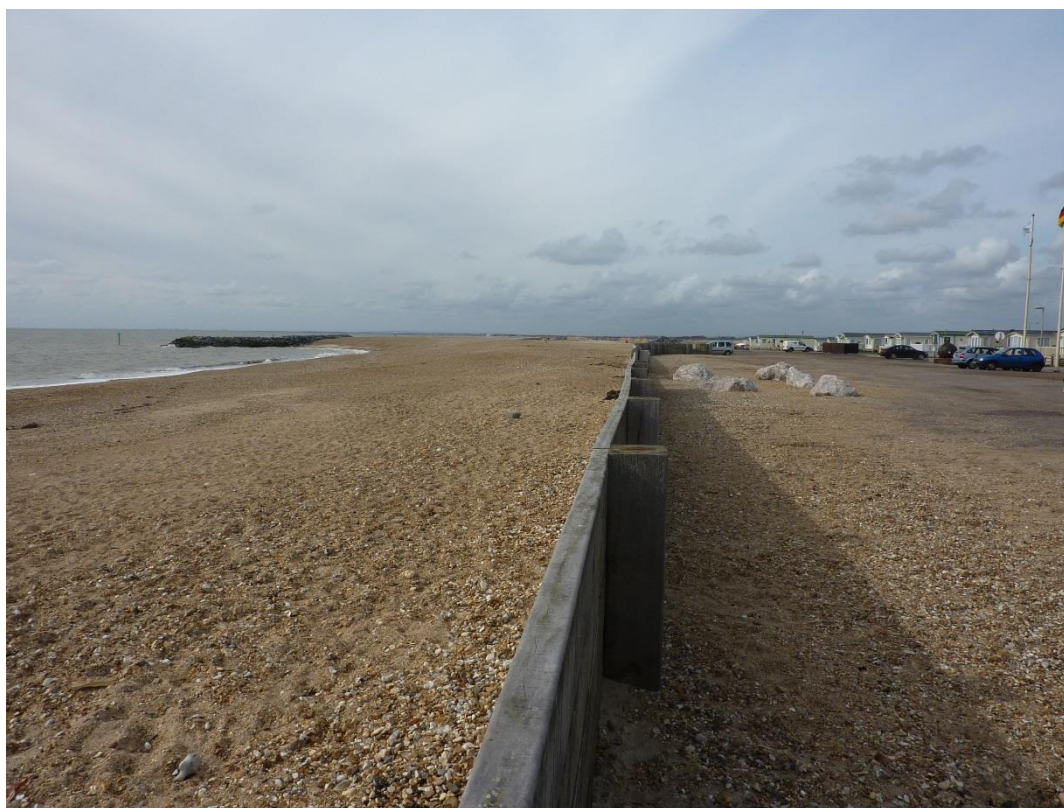
Figure 1-3: Wide shingle beach and rock groynes at Bunn Leisure complex
