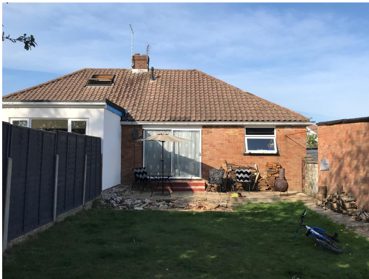
Photo 5: Rear of property
