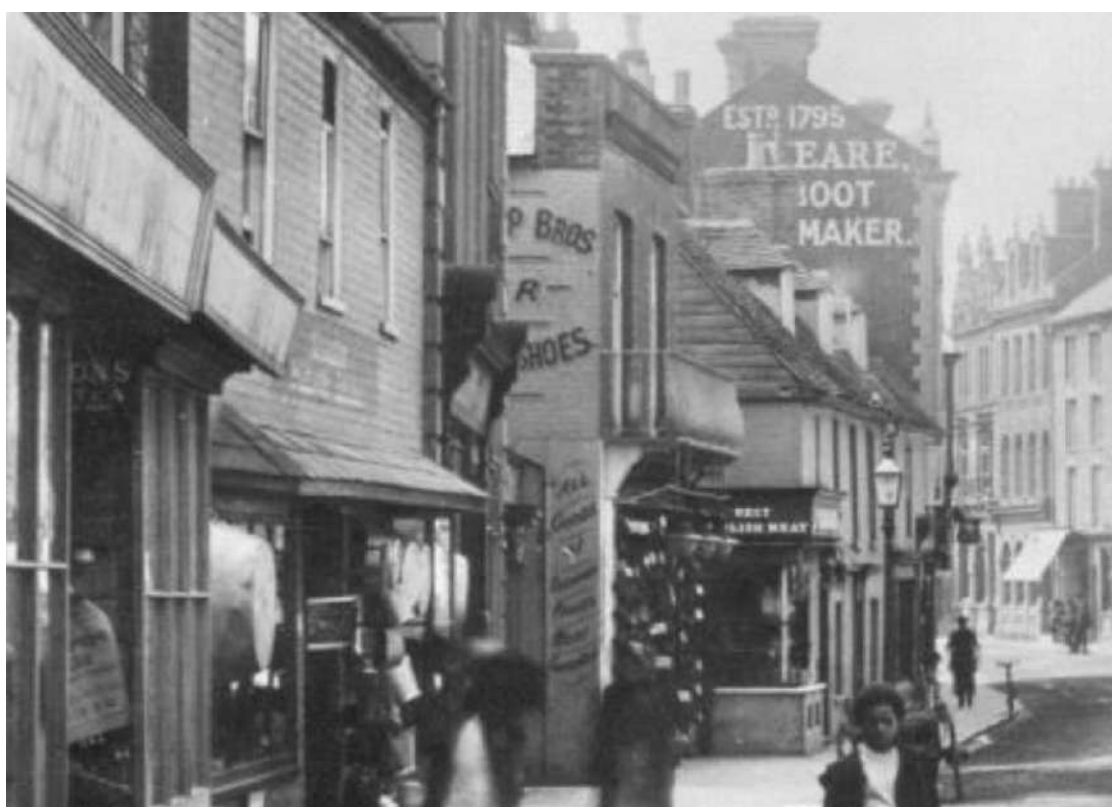
Figure 2: 14 East Street when it was used as a shoe shop, showing a balcony at first floor level.
