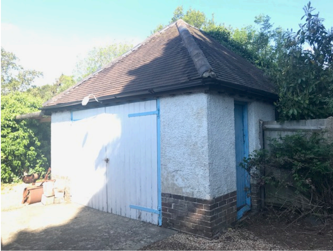
Figure 6. Garage set for demolition.
