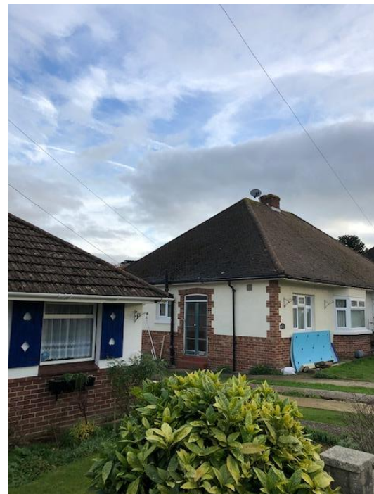
Street view of existing side elevation (North)
