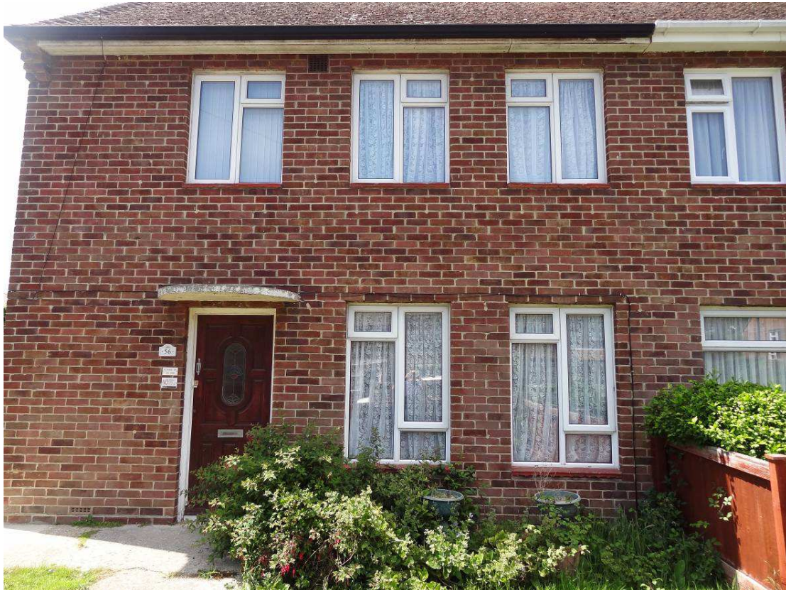
Photo 2 - Front (South) Elevation to No. 56 Kings Road
