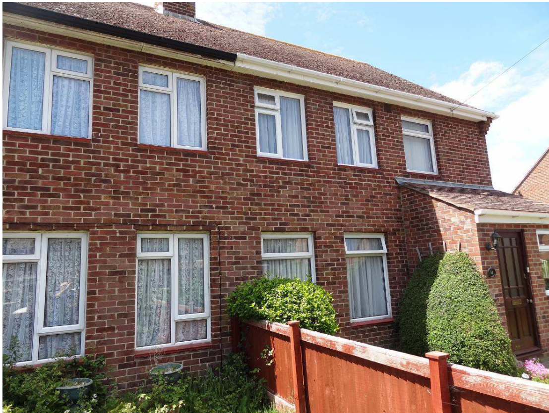
Photo 1 - View of Nos. 56 & 54 Kings Road.
