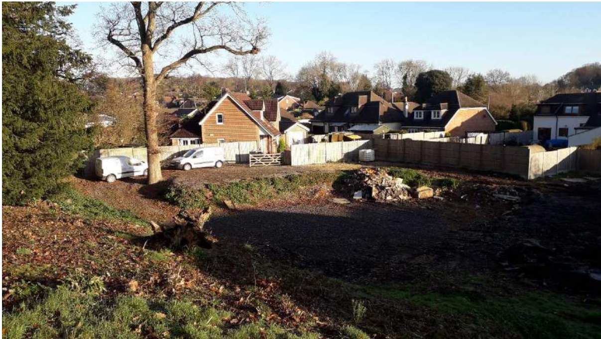
PLATE 3 – View of the site from the raised section facing north east
