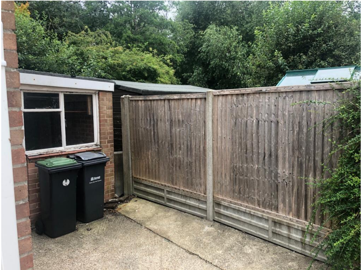
Photo 2: Front of storage room
