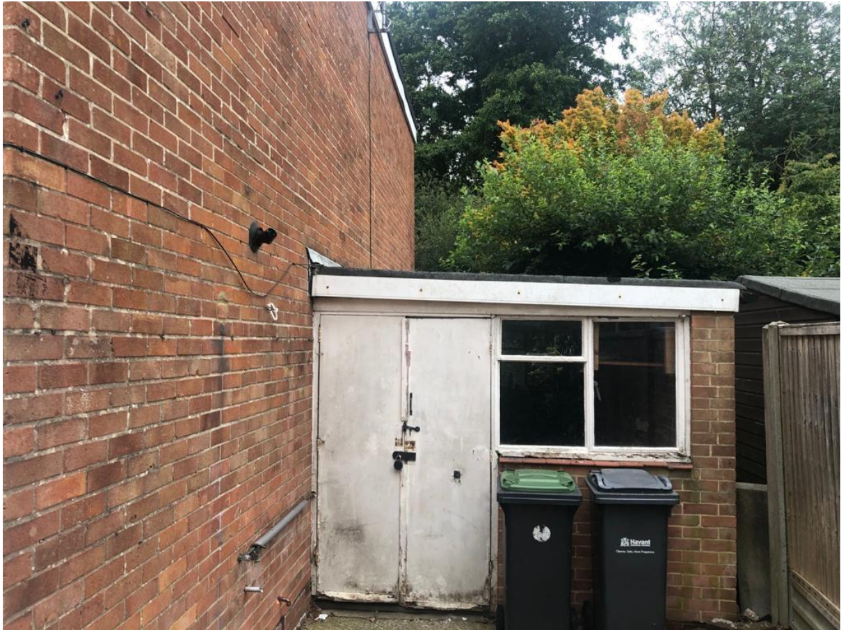
Photo 3: Front of storage room
