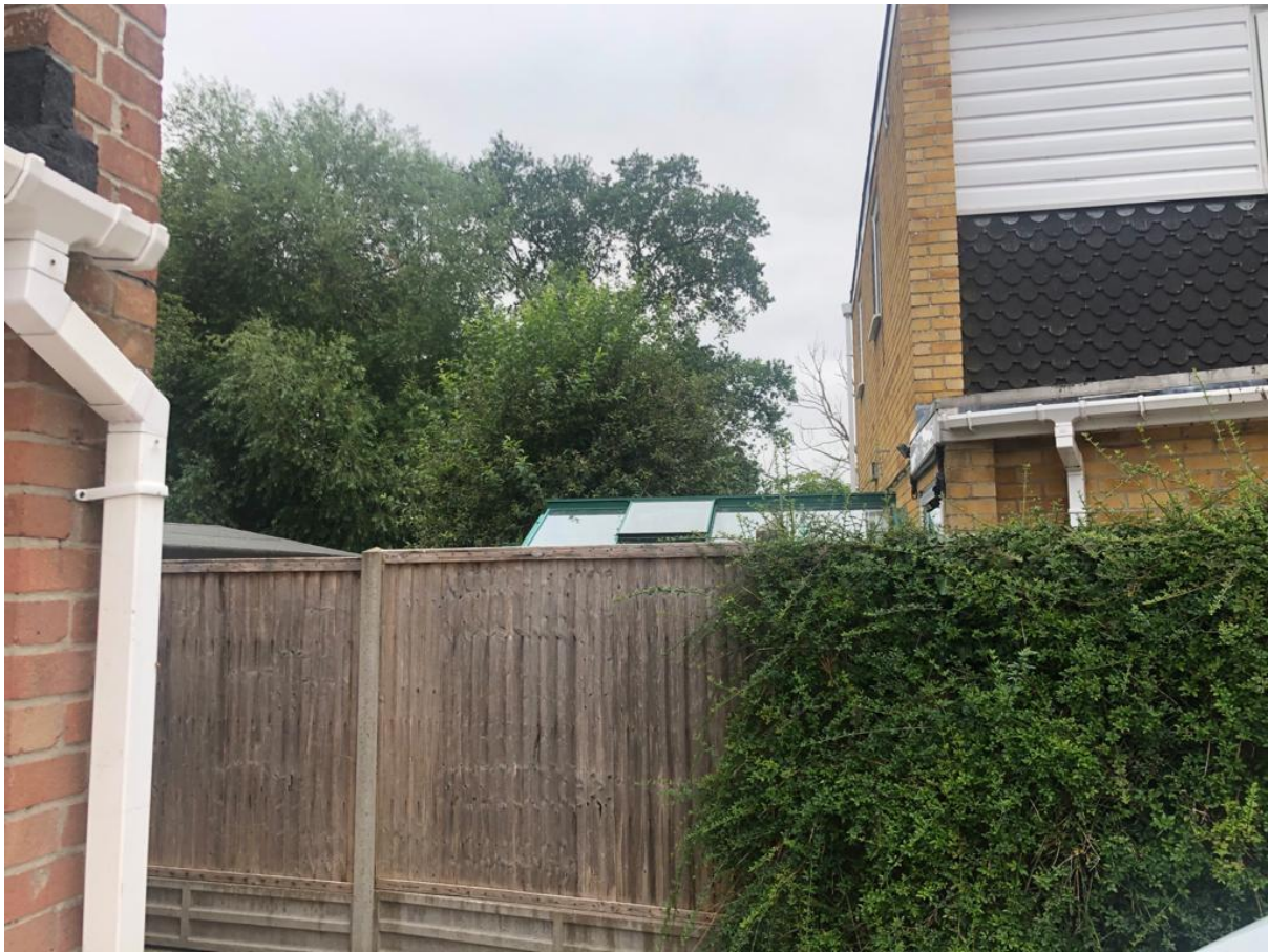
Photo 4: Side facing No. 32
