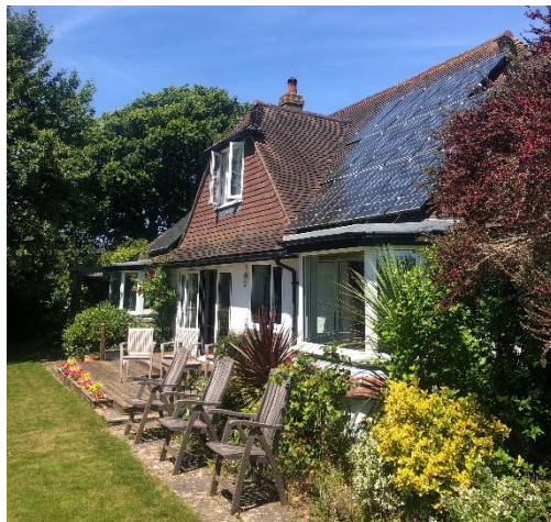
Figure 11: Existing rear elevation (South) from driveway
