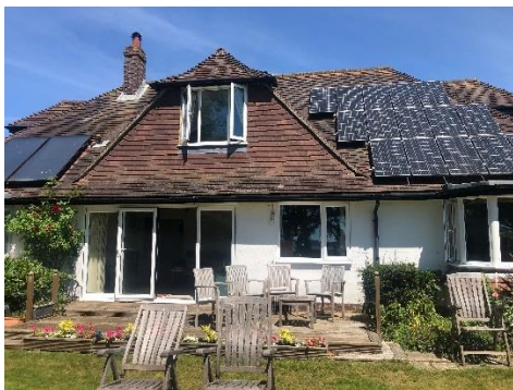
Figure 12: Existing rear elevation (South) from garden.
