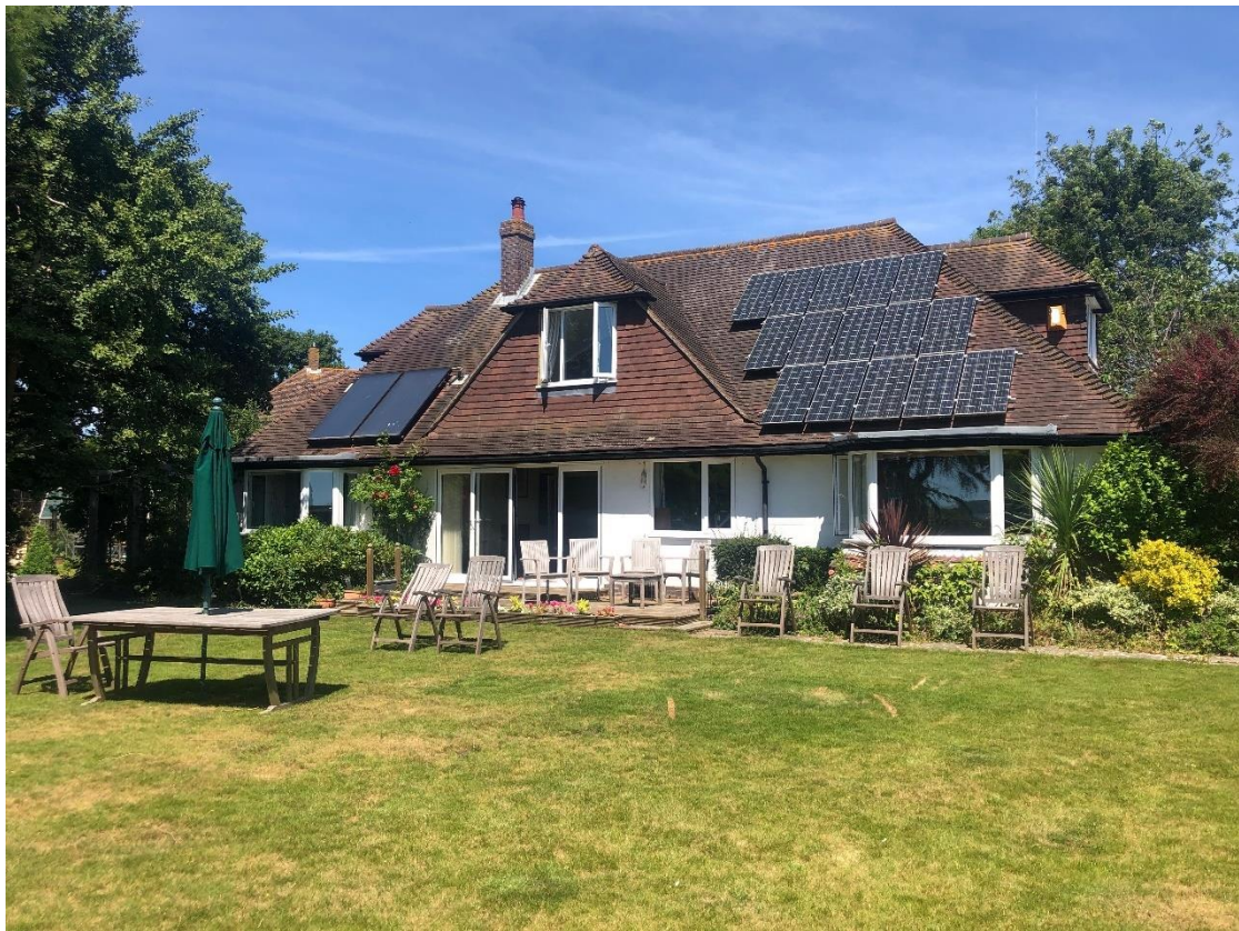
Figure 1: South Elevation of 67 Warblington Road
