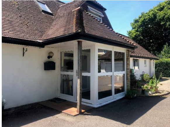
Figure 9: Existing front entrance
