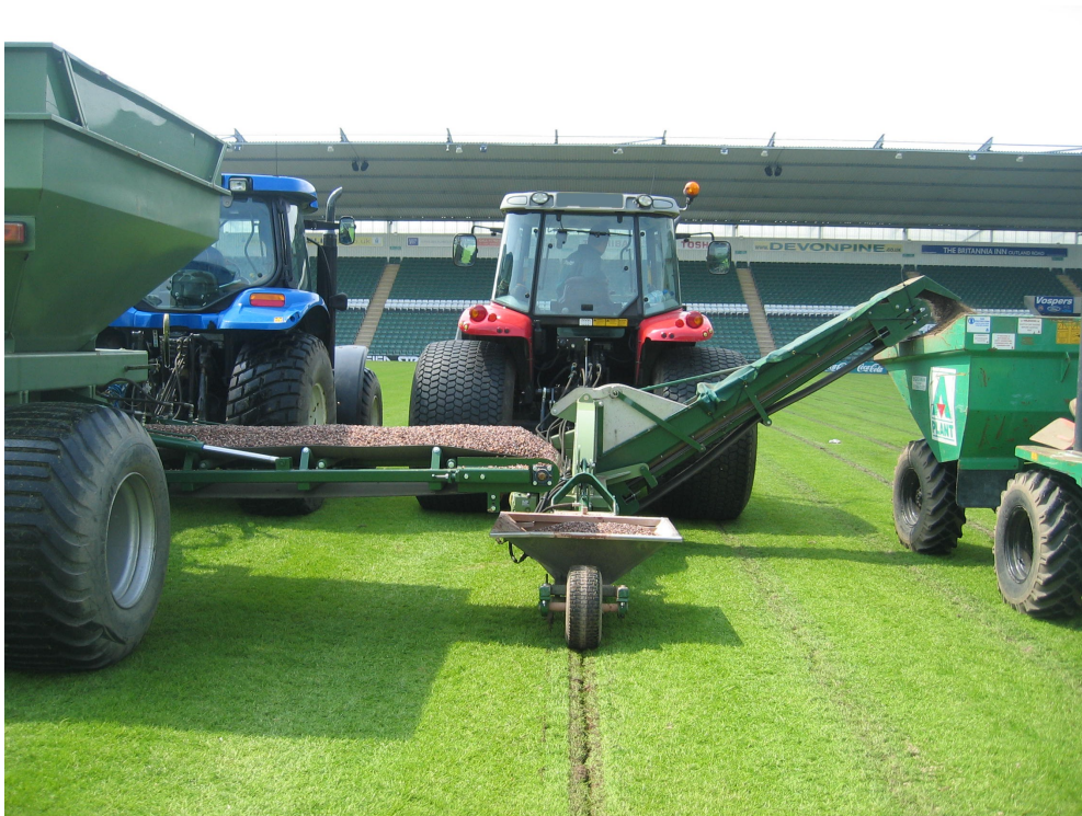
System 25 installing secondary drainage, Gravel Cart keeps hopper topped up
