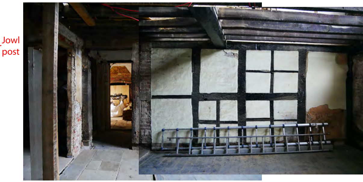
22. The central bay includes G9 and 10. There appears to have been doors on each side, that to west side altered, to the east blocked up. Evidence of fixed furniture to box frame. Wattle & daub was replaced with brick infill panels. Floor raised. Flags and floor boards are later finishes. Inner wall of G10 - side girt has racked and disengaged. Chamfers and run through stops to spine beam.
