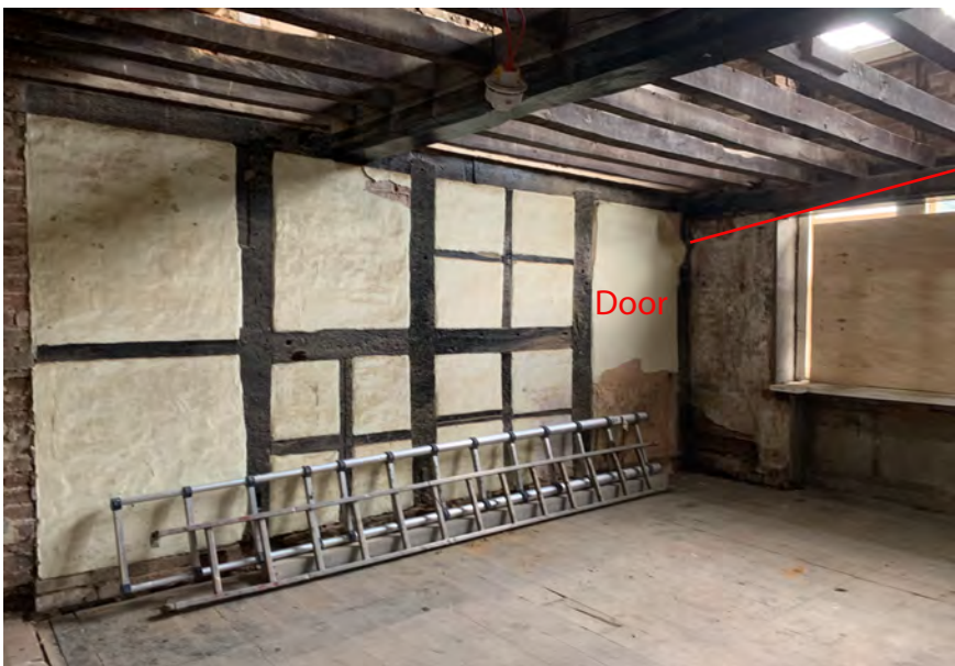
21. As per the former state but walls exposed, former door revealed and modern ceiling covering removed revealing joists.
