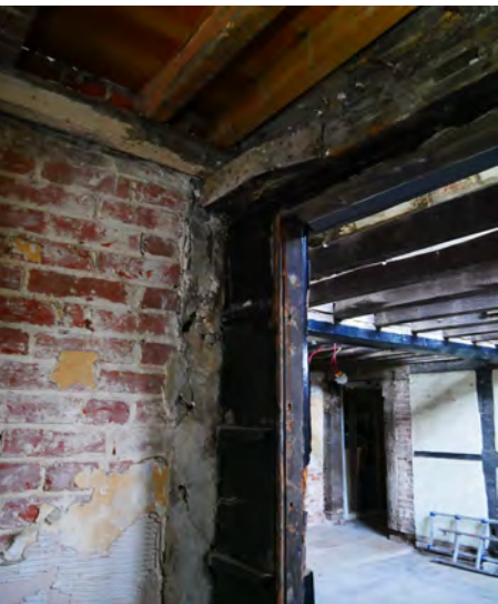
20. G7 - another former baffle entry. Blocked up and may have accommodated a stair/ladder to the first floor. This was used as an ensuite with tiled walls and floor and sanitary fittings.
