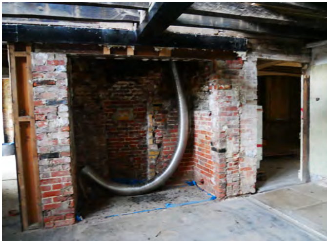
23. Used as an ensuite, tiled with wc & handbasin. Now removed & reveals past alterations to the brickwork, posts and an introduced steel RSJ. The Crossbeam above the door shows the original height of the room.
