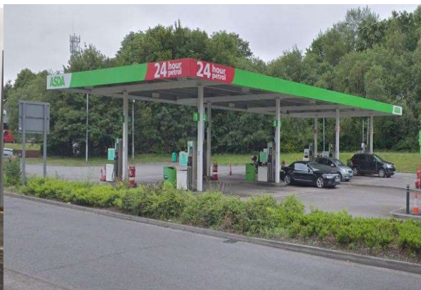
Existing South/East elevation to forecourt.
