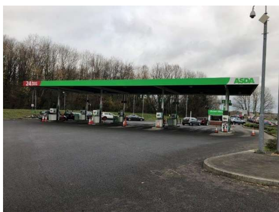
Existing West elevation to forecourt entry
