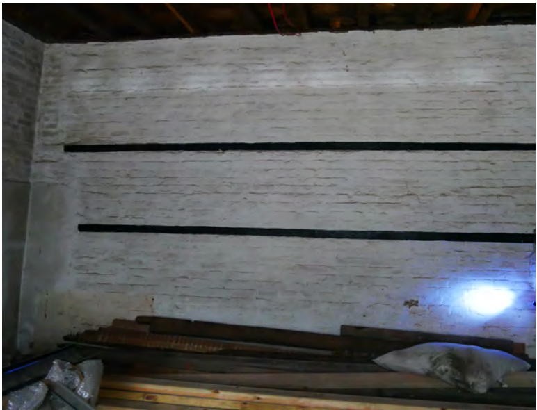
33. Inner face of east wall is more rudimentary in construction with timber.
