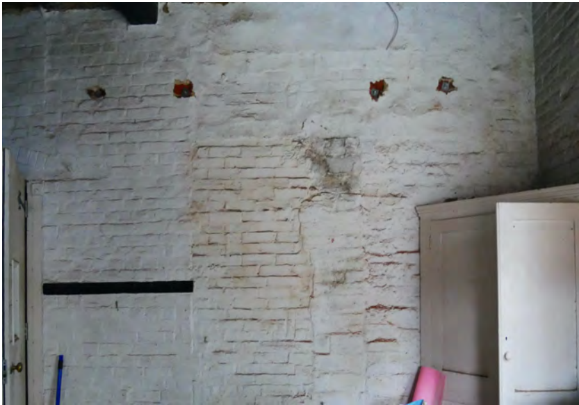
32. Inner face of south wall reveals a former door opening to G12 and a cambered arch to the door to G13. Bolts for new Floor to G11/12 noted.
