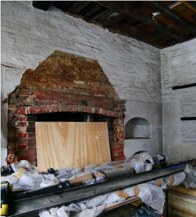
31. Inner north wall exposing brickwork to fireplace, higher arch to side indicating a possible doorway. Predominantly stretcher bond which could relate to the addition of the first cross wing. East and west walls are Flemish bond.
