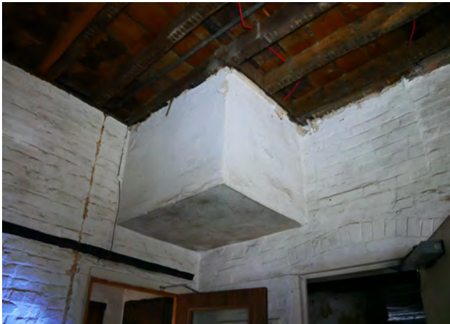
34. The bulkhead for the introduction staircase to the SW corner.
