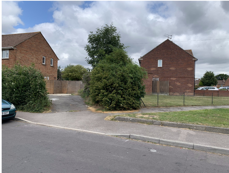
Site access - View from Selborne Avenue
