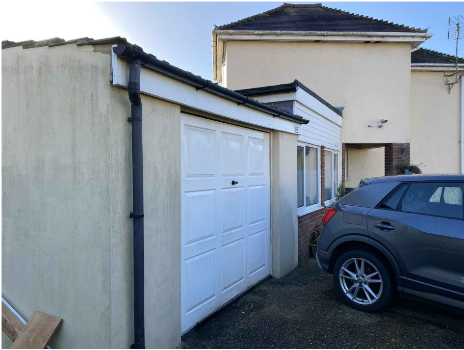
01 | View towards existing 'back door' showing various historic 'add-on' extensions and materials.
