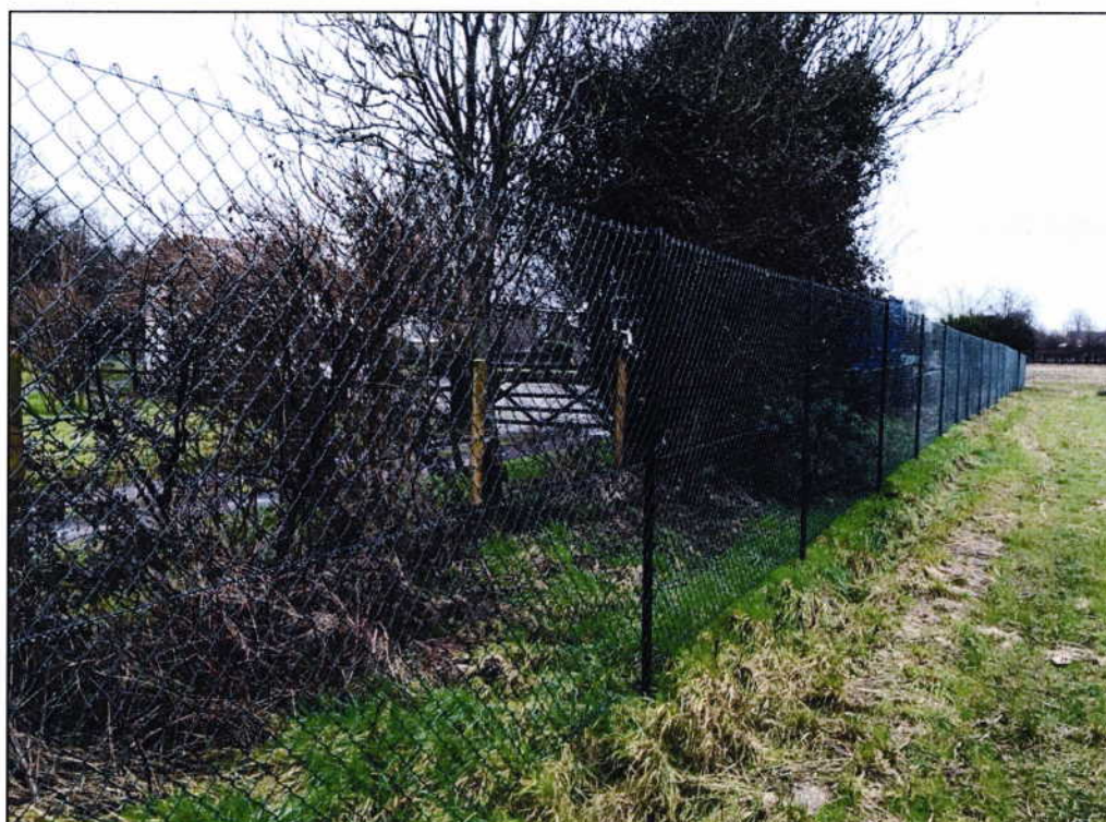
Chain-link on angle-iron uprights
