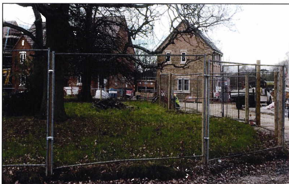
Weld-mesh panels on wooden posts
