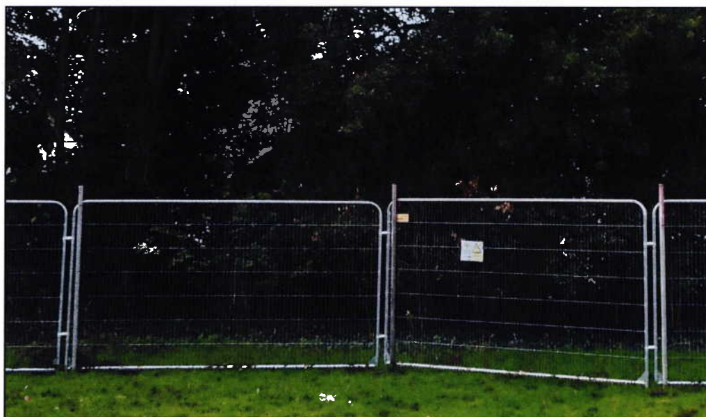
Weld-mesh panels on scaffold uprights
