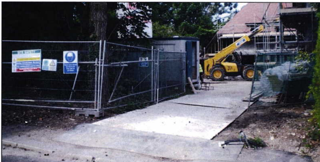
Vehicular ground protection trackway
