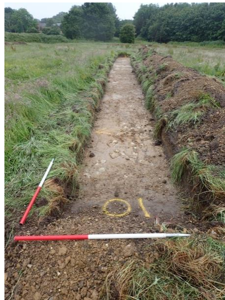
Plate 24: Trench 10, from the north-west
