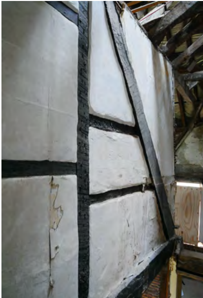
85. View of principal rafter, cross beam and east wall plate.
