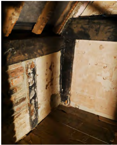
90. SE crnr of FF17 with cross beam, wall plate & possible former window.
