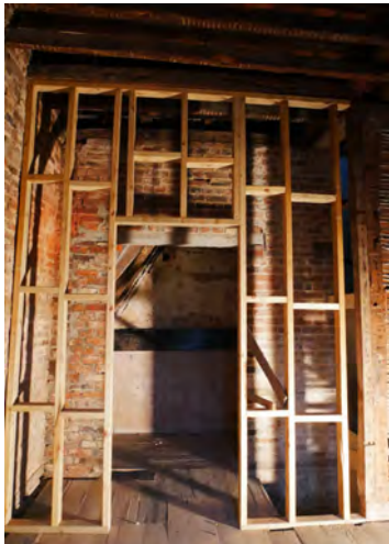
89. Partitioning in FF16 with FF17 used as an ensuite. Note the concrete RSJ. At a higher floor level than photo 88.
