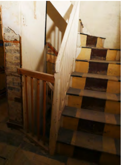
82. FF14 secondary Victorian stairs rising off landing. 1st flight rises from ground floor. Side landing also served FF17 but stairs removed.
