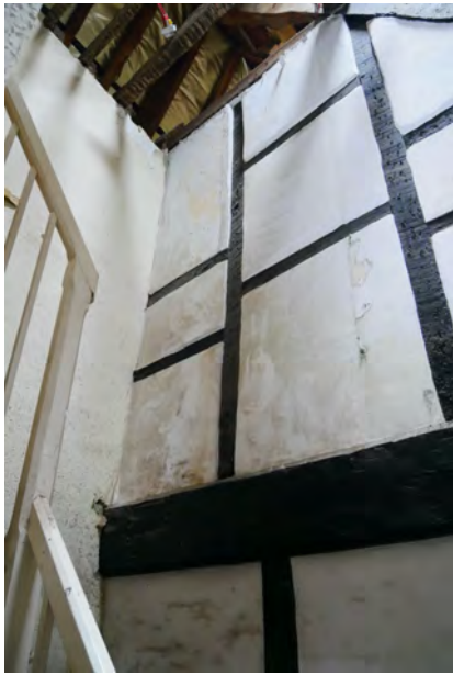
84. Cross beam & box frame rising up the stairwell wall. This would have been internal to the north 'ghost' bay.
