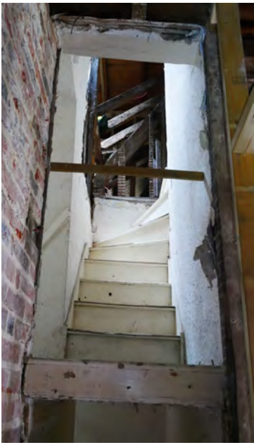
88. Stairs to attic off landing that also provided access to FF17. Taken from encroached area.
