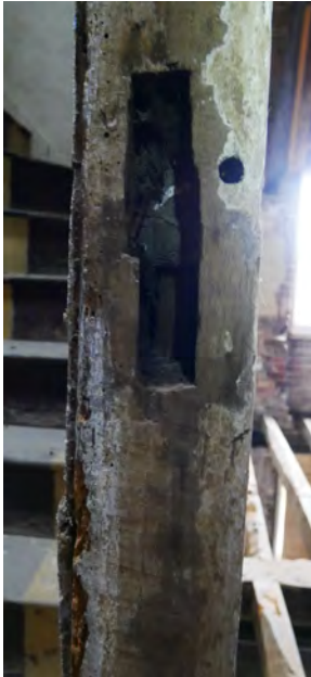
86. Evidence of missing rail. Underside of cross beam above shows position of former door to north bay.
